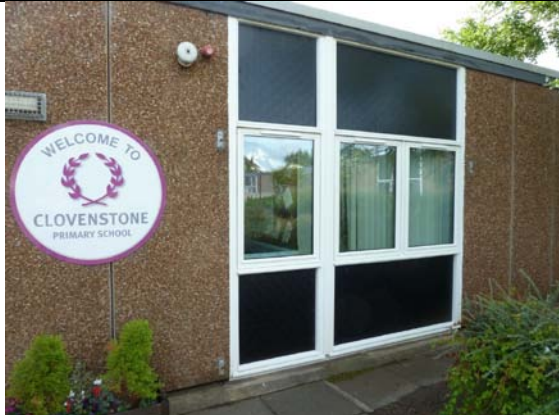
Clovenstone Primary School – New Windows
