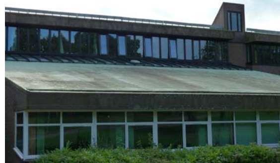
Balerno High School -New windows
