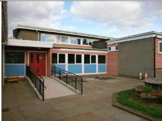
Nether Currie Primary School – Roofing, windows, doors, insulation, heating and electrical upgrade.
