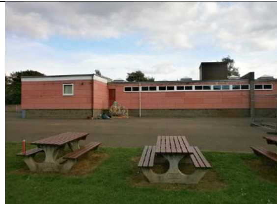
Nether Currie Nether Currie Primary School – Roofing, windows, doors, insulation, heating and electrical upgrade.
