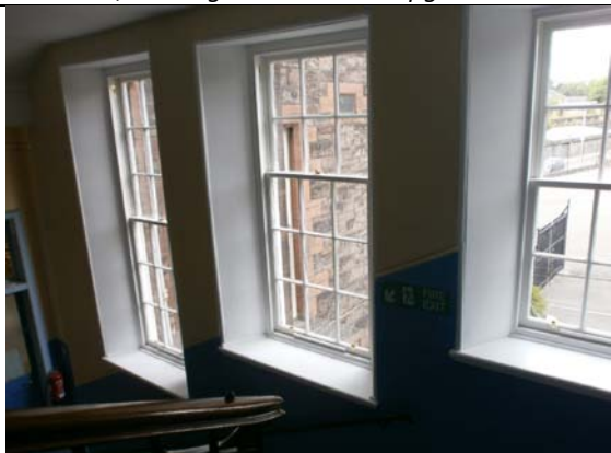
Abbeyhill Primary school – window refurbishment
