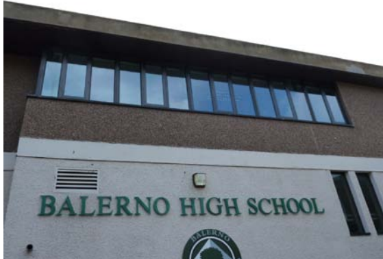
Balerno High School Replacement – New windows
